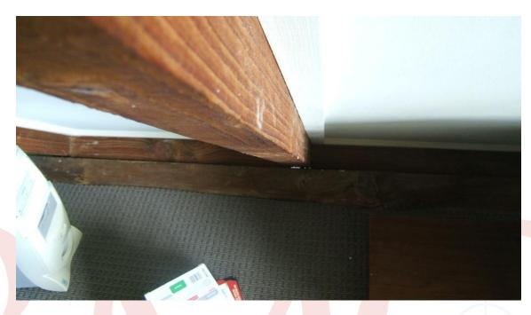
Rafter to Log Wall Fixing Separation (note daylight between rafter & log)
