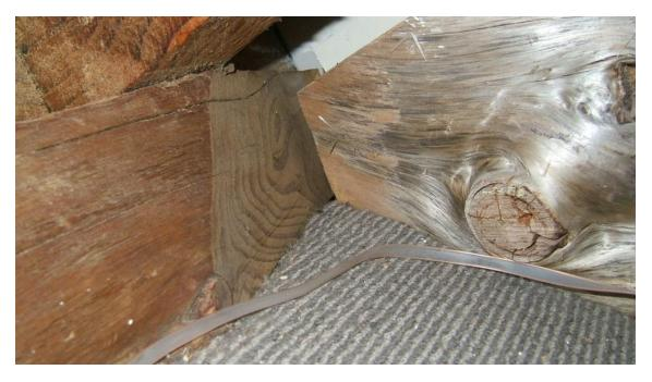
Rafter Fixing Separation & Log Movement
