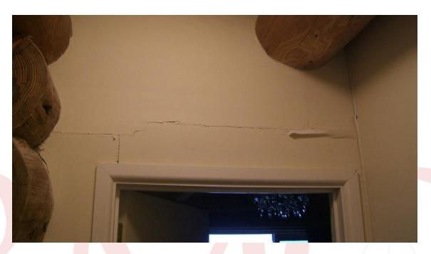
Internal Gib Board Wall Damage
